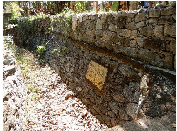
Figure 7 Uppukulam Thodu side protection
