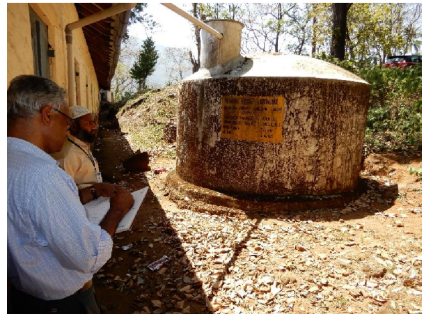
Figure 4 Rain water harvesting tank in Muthiyamala L P School
