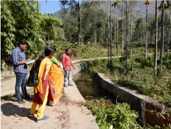
Mandokkuni check dam constructed in Mangavayal watershed
