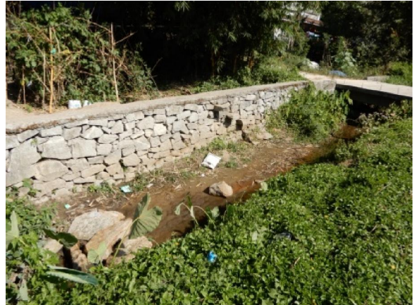
Side protection work in Mangavayal watershed
