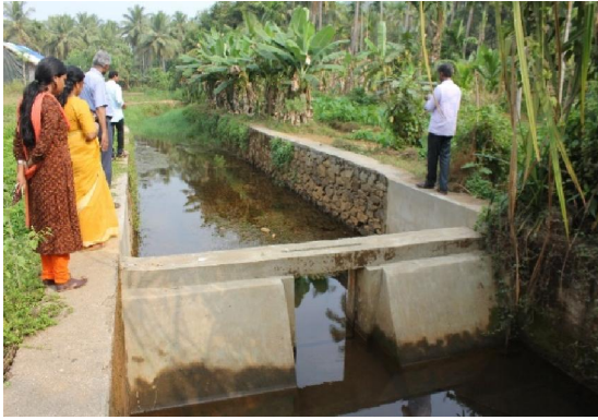
A VCB constructed across the stream
