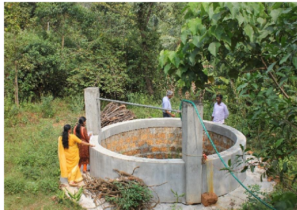
A newly constructed well in the project area
