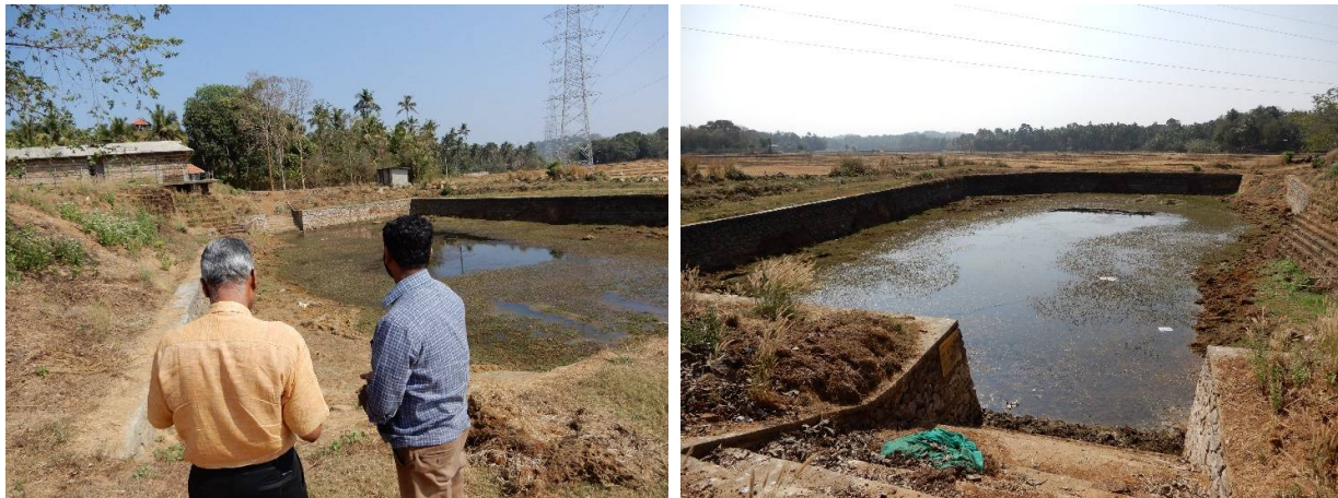
Figure 2 Renovated Pindarikkara Temple pond
