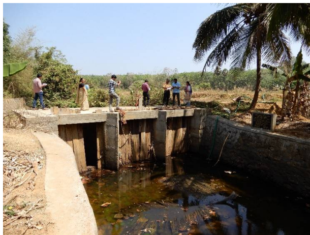
Fig 3 Kuthiramthodu side protection and shuttering
