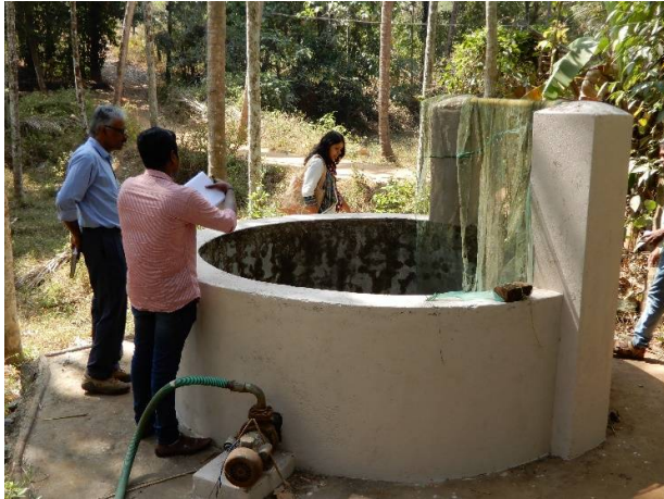
Figure 4 One of the open wells rejuvenated in Oduvoor
