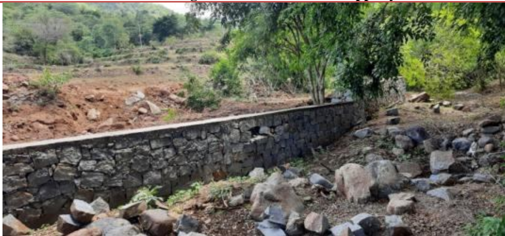
Kurumbamutham Thodu Side Protection
