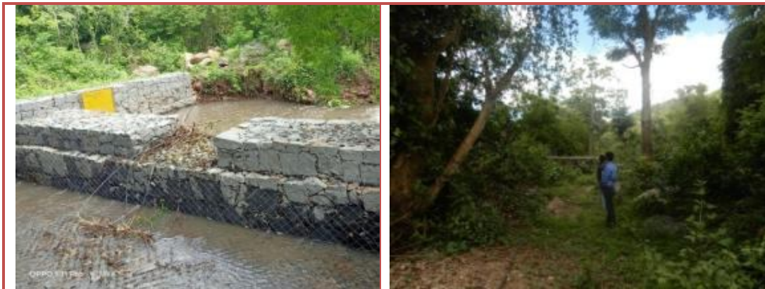
Konamkuthipallam Gabion structure
