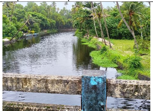
Chennavelipozhi- Janapathi thodu renovation
