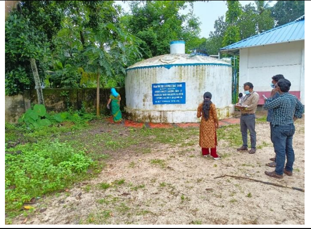
Rain Water Harvesting at St.Antony's high school, Kokkothamangalam
