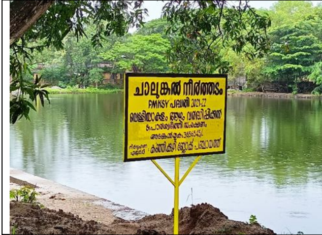
Pond renovation at Velliyakulam
