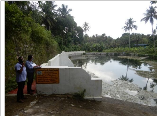
Pond renovation at oorgam, Aratupuzha watershed, Cherpu Panchayath
