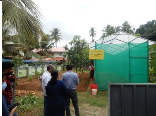
Rainshed work for SHG at KuchhuMuhummed house
