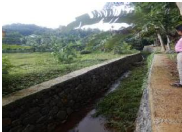
Side protection at ParakadavuVayal thodu
