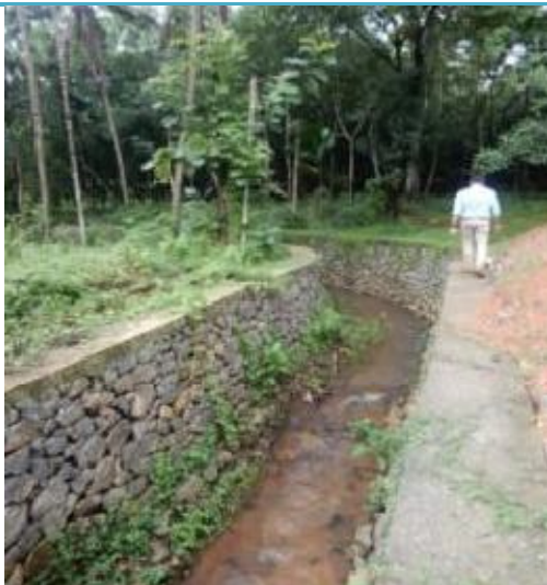
Side protection of Alathur stream
