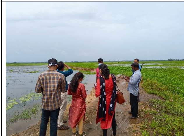
Kudivellari A padasekharam thodu deepening and bund construction
