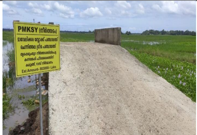
KandalkaripadamKalukku Ramp Construction
