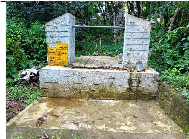
Renovation of Charakuzhy public well
