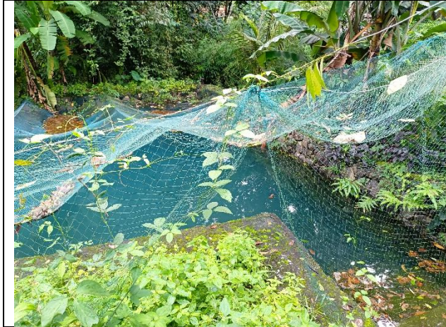
Renovation of Puthussery Dharmasathra temple pond
