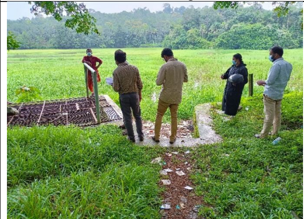
Renovation of palamukku natural spring and side wall stabilization
