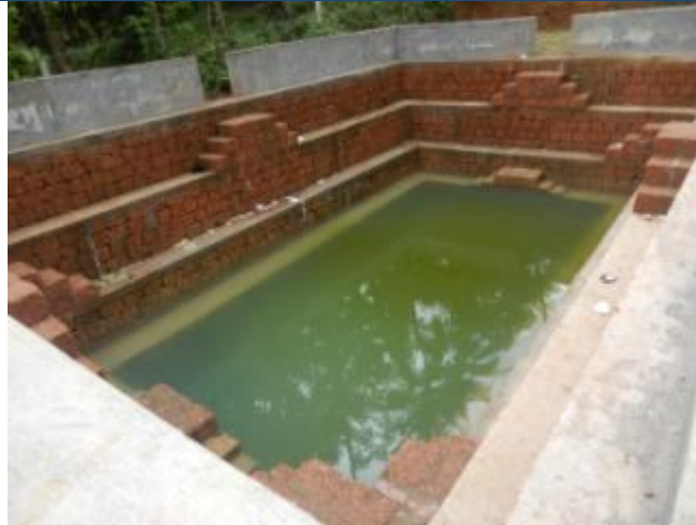
New pond construction at Madathil watershed
