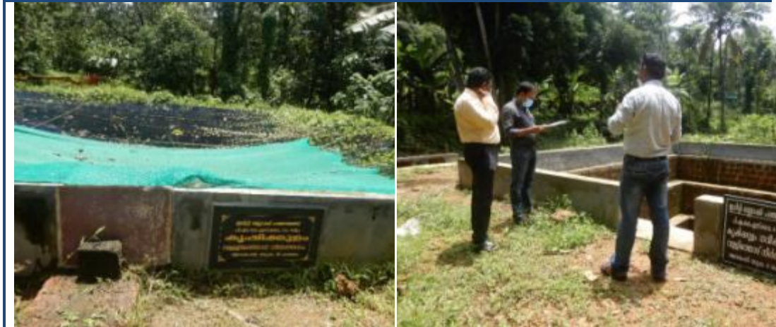
New pond construction at Vallithode watershed
