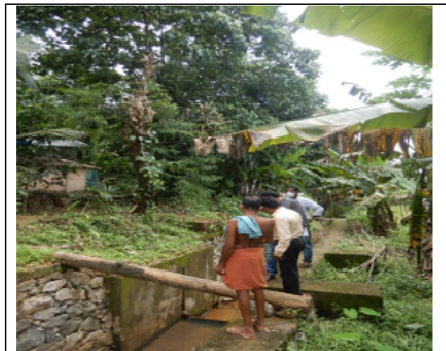
Check dam with side protection At Ayirakulam
