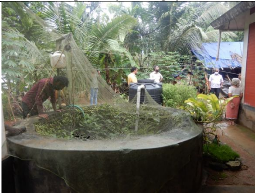
Rain water harvesting structure at Balakrishnan house
