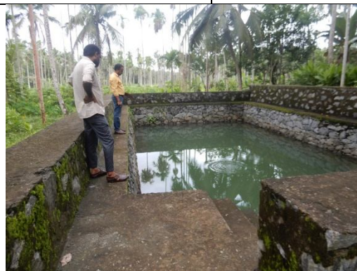
Pond renovation at Mandokandi
