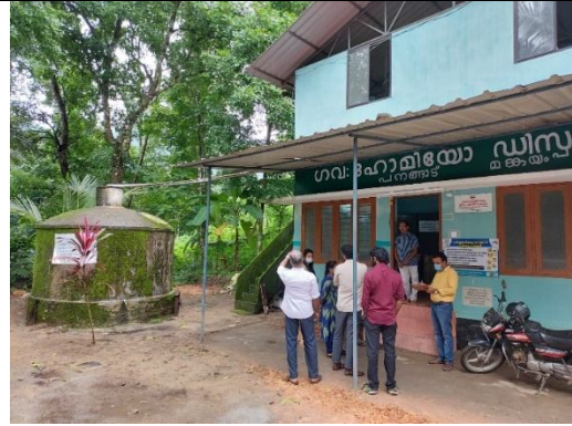
Rain water harvesting tank at Govt. Homeo Dispensary, Mangayam
