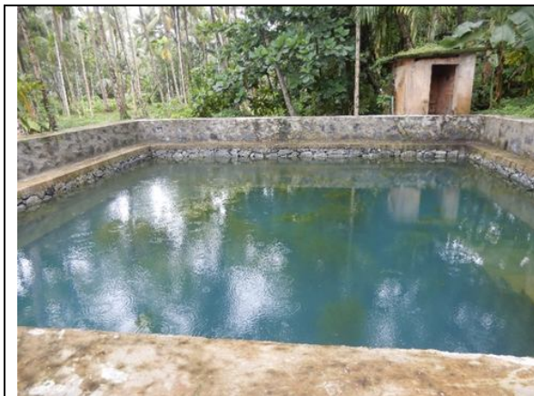
Renovation of KandothThazheKulam
