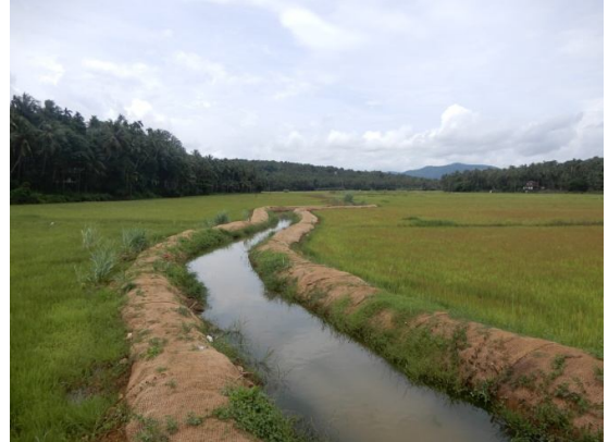
Kuttoor thodu Side bund stabilization with silt removal
