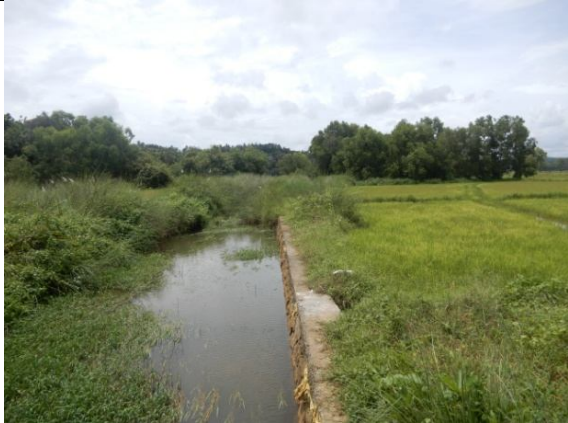
Side wall protection at Kuttoor thodu watershed
