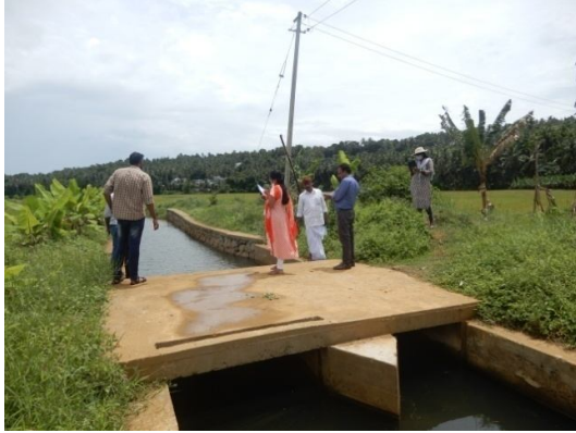
VCB at kuttur thodu watershed near Fasiliyar road
