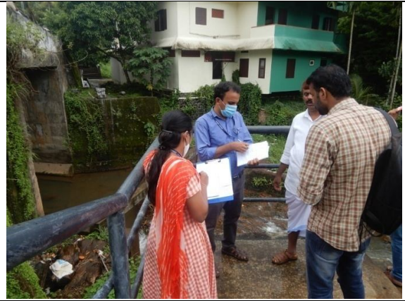
Vettuthodu Side protection wall
