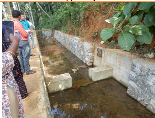
Stream bank side protection
