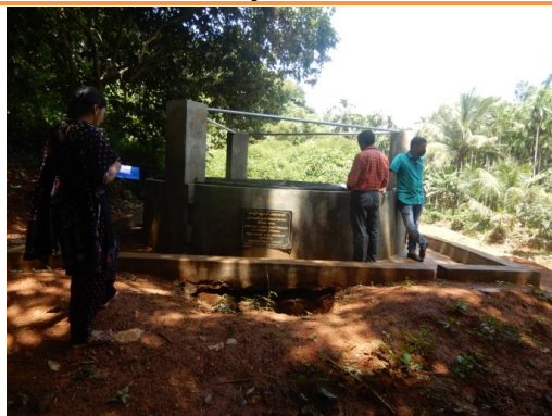
Chathankulam well construction
