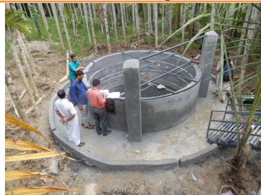
Pandikkad well construction
