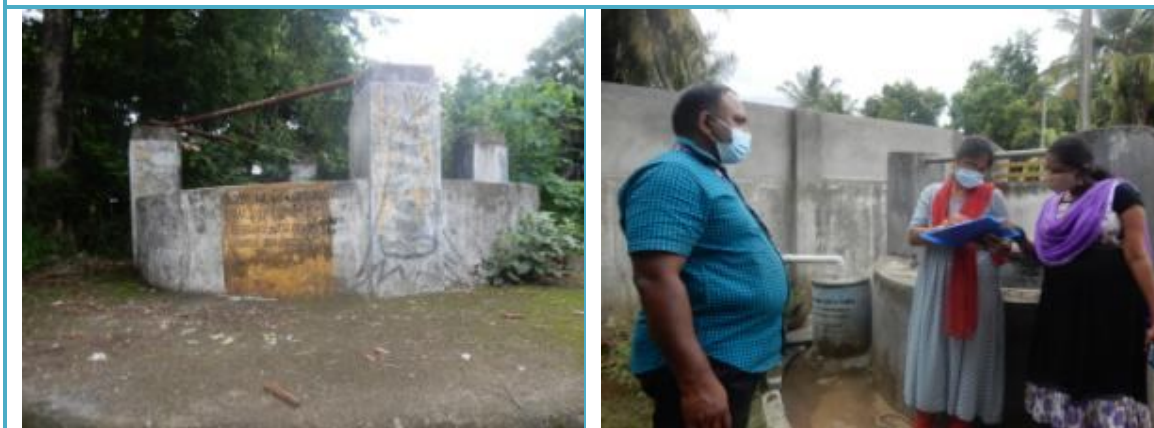
Public well renovation
