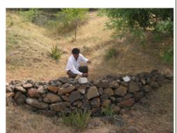
along acontour line. A contour line is a line which joins together points of the sameelevation. Digging a trench along such a line increases the chances of retainingrunoff for a longer period of time within the trench. It is also true that if trencheswere not along the contour, such digging could actually increase the possibility ofsoil erosion.
