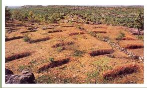
the spacing between the rows may vary from 3-5 m. The chances of breaches of SCT are less as compared to Continuous Contour Trenches. Over time, experience of watershed programs has shown that it is better to stagger the digging of contour trenches. This is because it has been found
