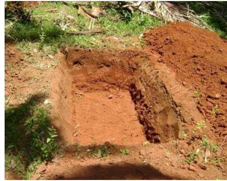
Rain water Harvesting Pit
