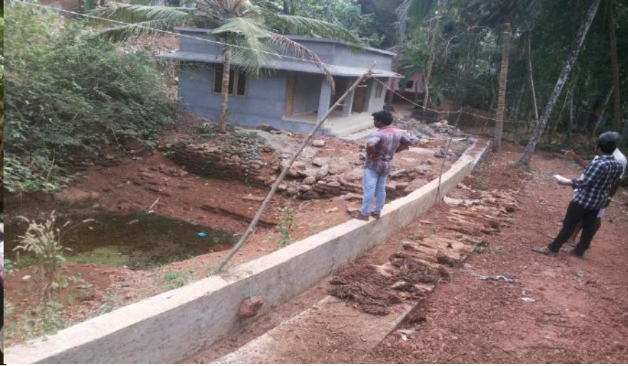
Chola kulam repairing
