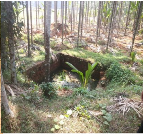
Vallikkadu pond renovation
