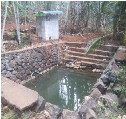
Parapurathmoola pond renovation
