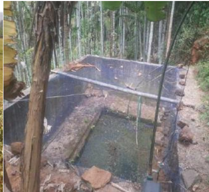
Kokkulangara pond repairing
