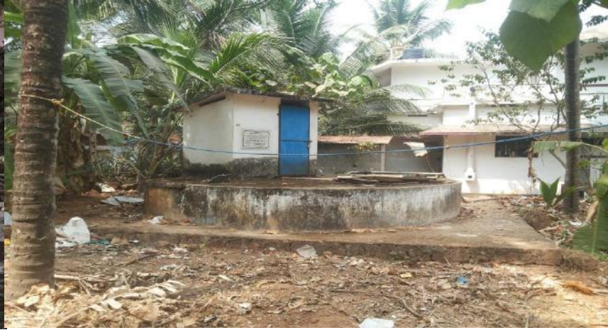
Mulamkunda well renovation
