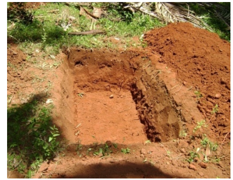
Rain water Harvesting Pit
