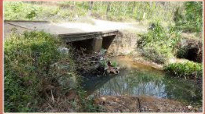
The waterflow is blocked due to waste filling
