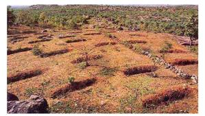
ContourTrenches are adopted. The length of the trenches is kept short around 2-3 m and the spacingbetween the rows may vary from 3-5 m. The chances of breaches of SCT are less as compared to Continuous Contour Trenches. Over time, experience of watershed programs has shown that it is better to stagger digging of contour trenches. This is because it has been found that invariably errors
