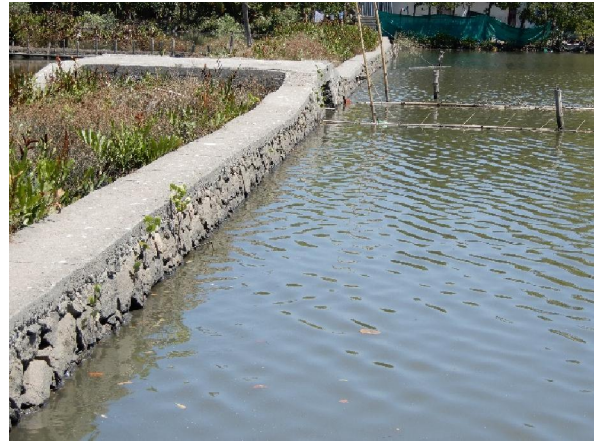
Thamaravattom Vadakkumbhagam side protection and sluice
