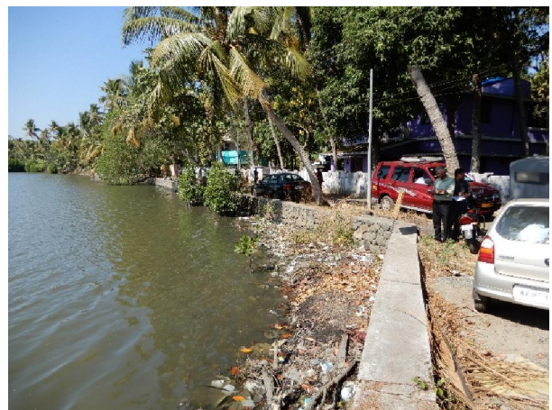
Strengthened outer bund of Ayyampilli Paadasekharam
