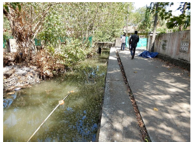
Side protection and culvert near Union U P School
