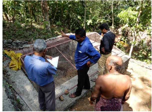
Spring protection and renovation in Nedungazhi watershed
