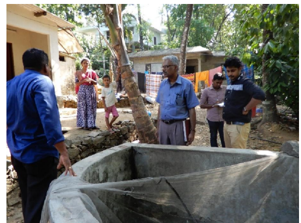
Newly constructed well at Aaniyilappu
