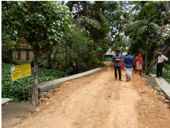
Pipe Culvert constructed at Kandamkulam
