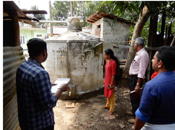
Rainwater harvesting tank in one of the households in Kuttamangalam watershed
