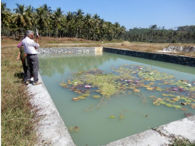
Farm pond constructed in Thrikkaipetta watershed
