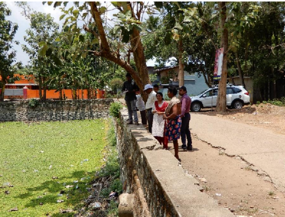
Renovated Nenmani Chira pond
