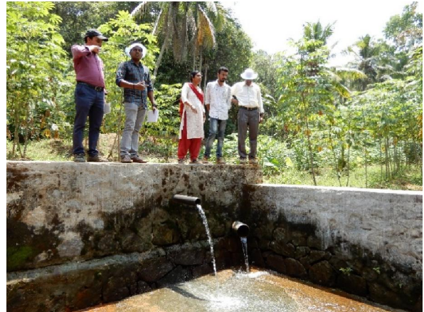
Perennial spring protection at Anjaam Poyka
