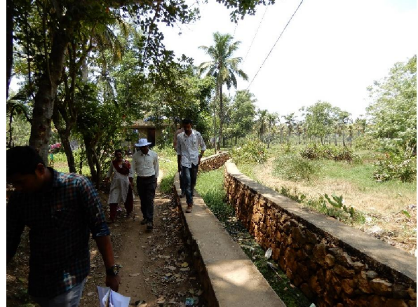
Side protection work of Moozhiyil Thodu in Mylakkadu watershed
