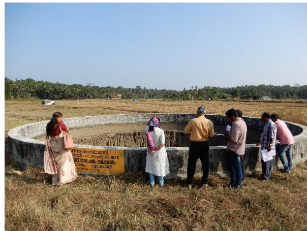
Figure 3 Renovated Palakkal Thazham well
