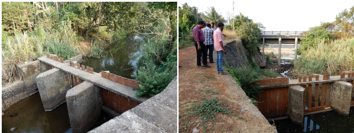
Figure 2 Shutter constructed at Chittappura near Puliampattakayal
