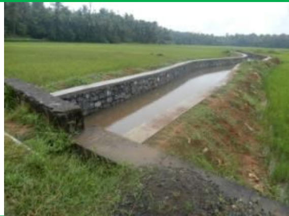
Kothakulam thodu side protection
