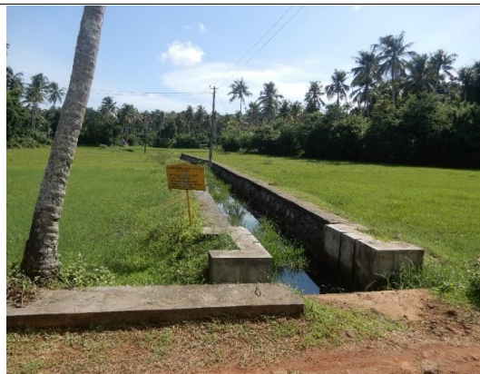
Kanjirapullam thodu Sluice at Kombsthu Kadavu
