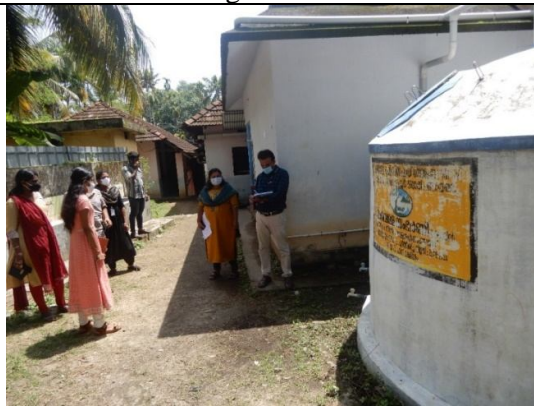
Rainwater harvesting tank, GUPS school, Velivattom
