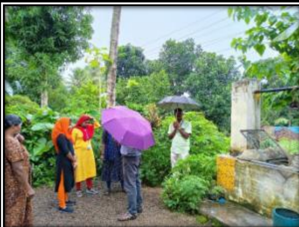
Well construction of Richel at Kunnampalli
