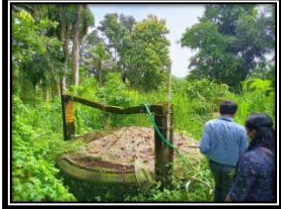
Ground water recharge at BDO office
