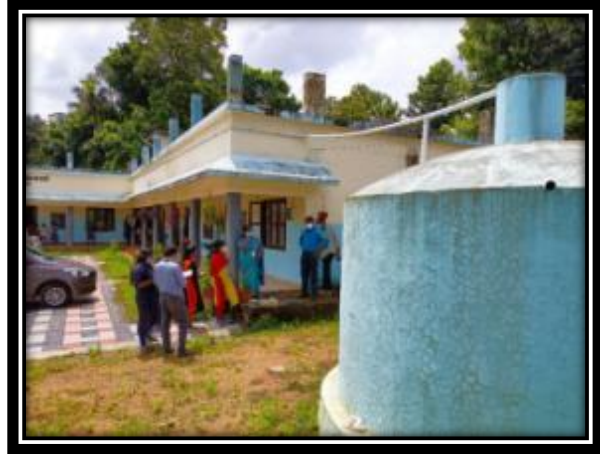
Rainwater harvesting tank at Govt. U.P. School, Velluthuruthy
