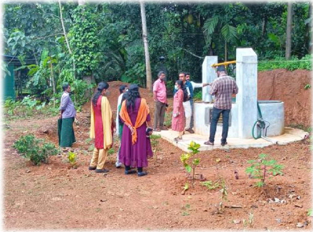
Thaleeradi Harijan welfare department well renovation
