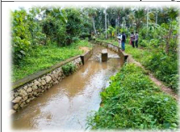
Parayattuvayal – Alakkukadavu check dam
